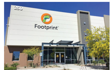
Sustainable technology firm Footprint is using new manufacturing processes at its Gilbert, AZ facility (above) to revolutionize the production of single use plastic cartons, cups, trays and straws, among other items. (Photo: ACA)
